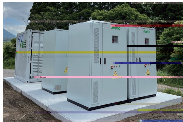
Fig. 2 Jinko ESS 215kWh DC Blocks
